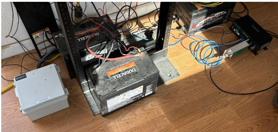
Figure 6-4 Indoor Wayside Contention System Installation
