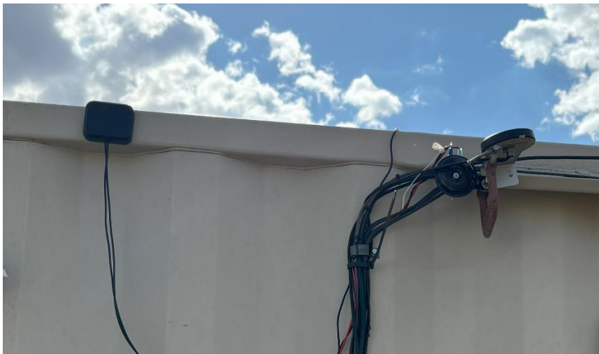
Figure 6-5 Indoor Wayside Contention System Cellular and GNSS Antennas
