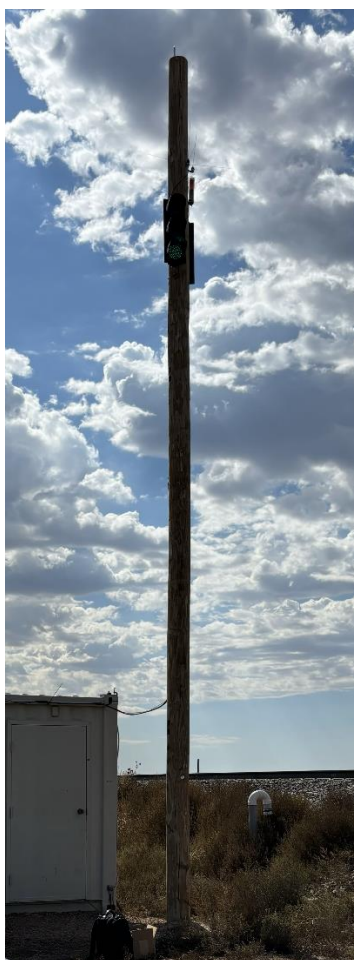
Figure 6-6 Indoor Wayside Contention System RF Antenna
